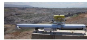
Figure 6. IBIS-M installation at Çollölar.
