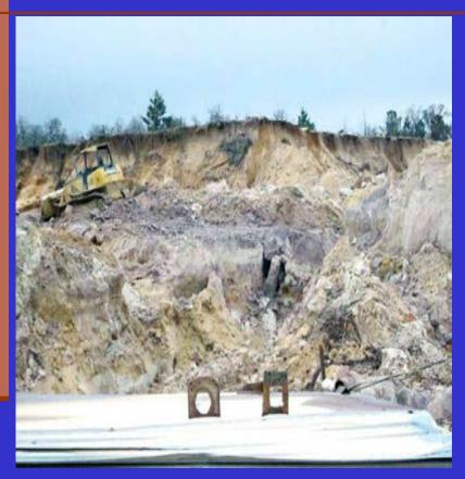
A water cannon operator walked to the edge of a 27 foot deep trench when the bank of the trench collapsed engulfing him.
